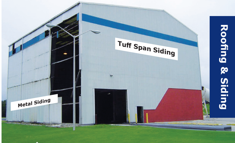
At Waste to Energy facility, Tuff Span roofing and siding (on end wall) were undamaged by Hurricane Charlie's 145 mph winds. Corroded metal panels (on side wall) were damaged or blew off.
