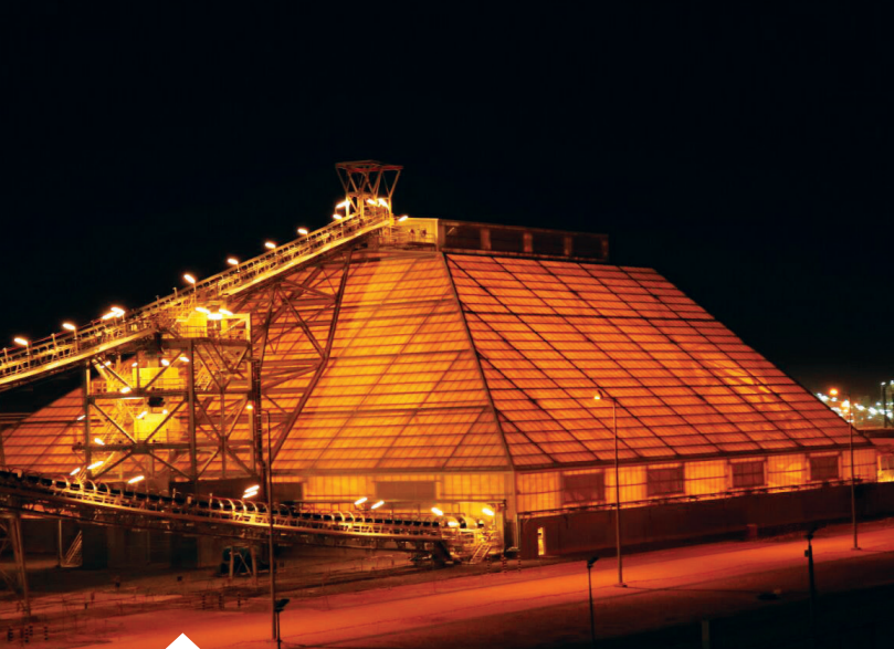
Tuff Span translucent roofing & siding at phosphate storage facility.
