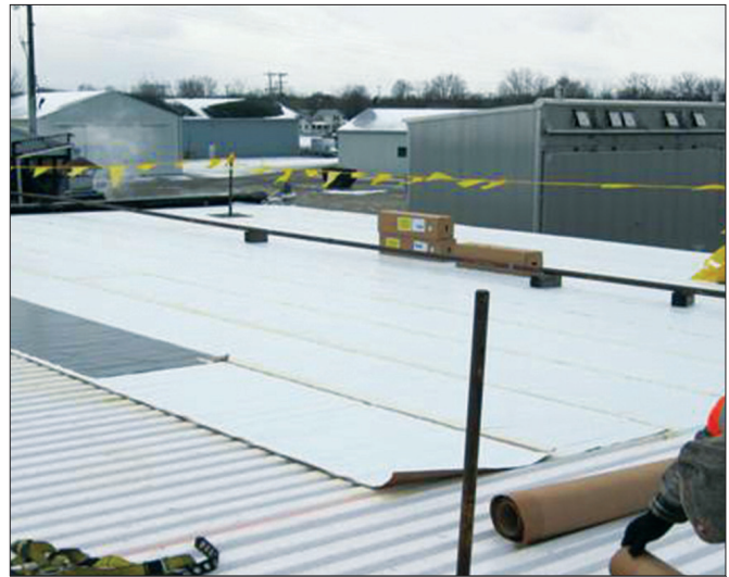
Corrosion resistant Tuff Span Roof Deck is a suitable substrate for either single-ply or built-up roofing
