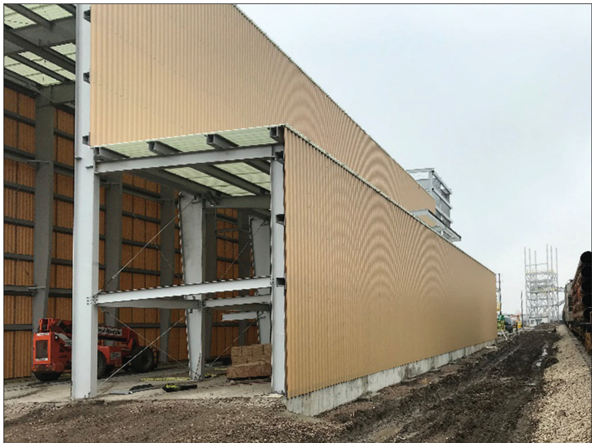
Tuff Span 8F6 purlins and girts on a fertilizer storage facility.
