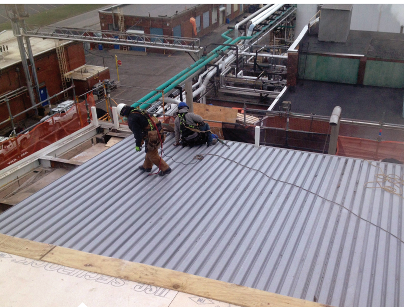
Tuff Span roof deck installation at chemical plant
