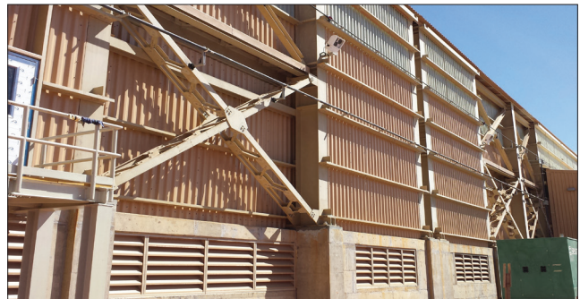
Tuff Span Louvers, Beams & Cladding at copper mine
