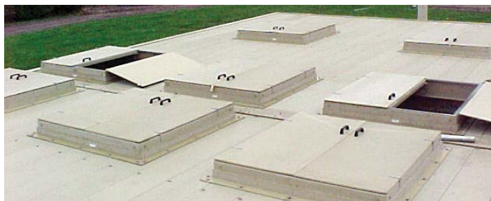
SureGrip beam-supported tank cover system and access hatches Sedimentation Basin
