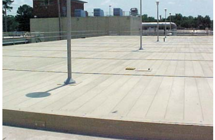
SureGrip beam-supported tank cover system Sedimentation Basin
