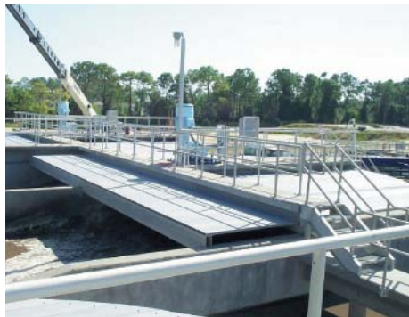
SureGrip beam-supported splash cover Racetrack Aeration Basin
