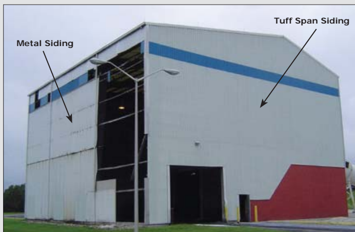
Above: Metal siding at waste-to-energy plant was completely blown off or damaged while the adjacent Tuff Span siding and roofing withstood the extreme winds.
