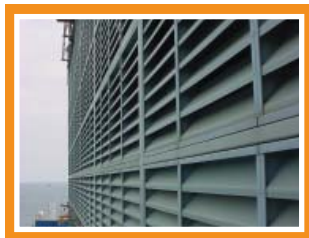
Enduro FRP louvers on an offshore platform off the Gulf Coast
